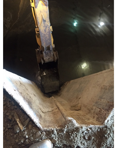
Final scraping of sheet pile walls
