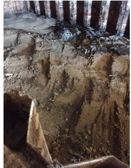
Cleaning of Cells 1 and 3
