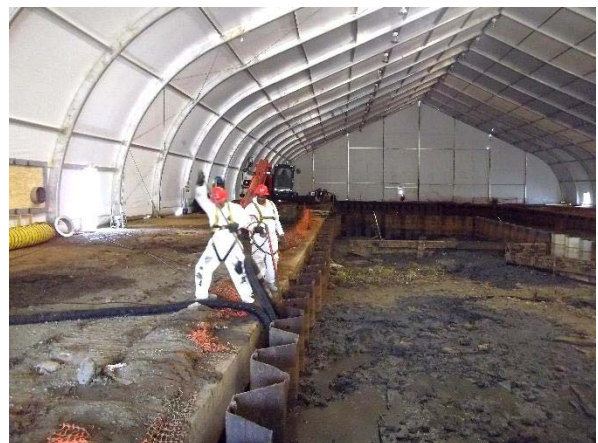
Removal of material from annular space
