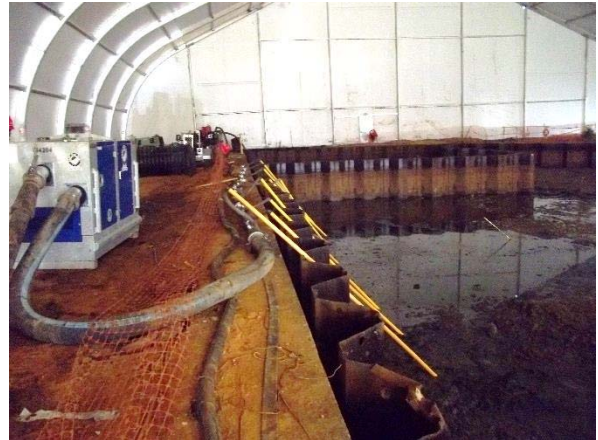
"Well Point" dewatering system
